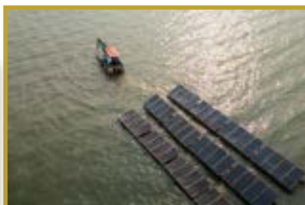
Floating solar photovoltaic system
